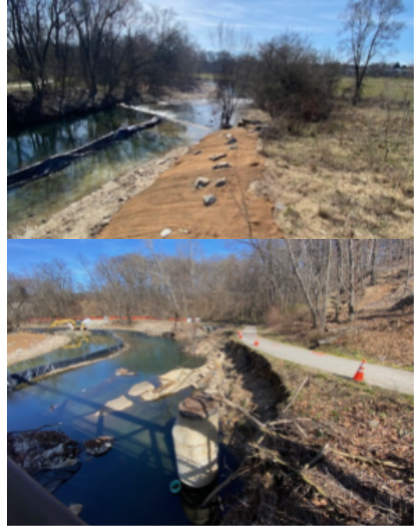
A view from pedestrian bridge of work area
